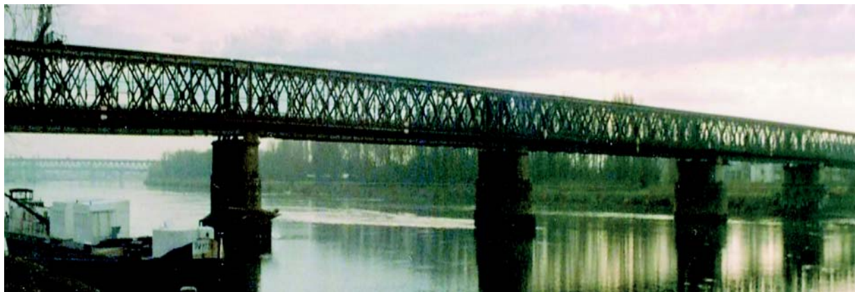
Fig. 5 Old Bridge in Bratislava
