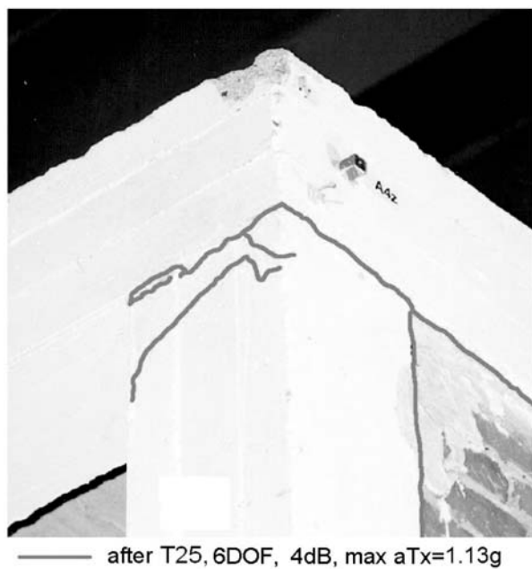
Fig. 9 Cracks in critical sections of R/C frame at the end of test - top of the frame
