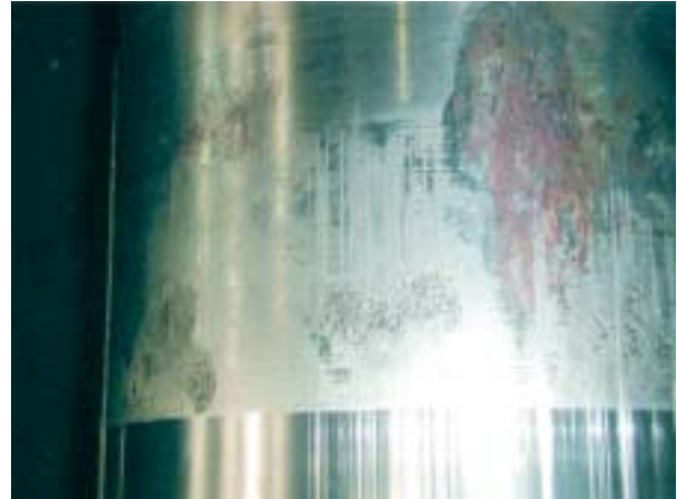
Fig. 12 Deep and shallow pittings on the functional surface of the rod
