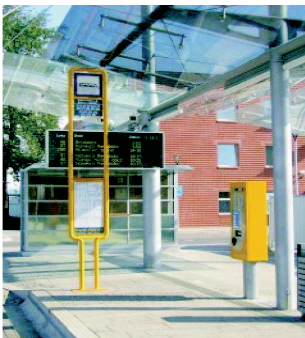
Fig. 5 Refuges and corridors must be designed with regard to carrying capacity and safety
