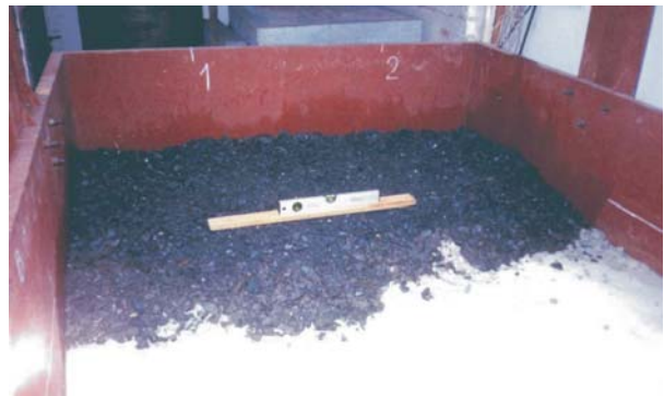
Fig. 4 Building of the sub - base layer of thickness of 150 mm
