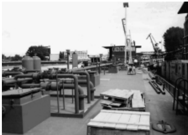
Obr. 6 Prestavba lode Fig. 6 Rebuilding of the ship
