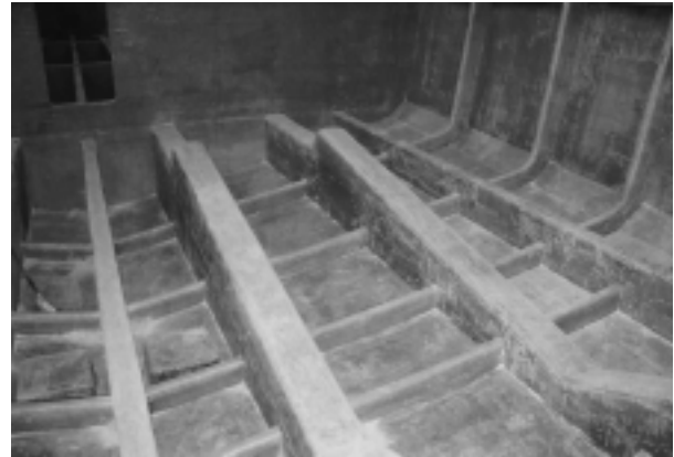
Obr. 3. Chrbtice a lôžka motorov v strojovni Fig. 3. Keelsons and engine seating in engine room
