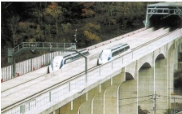
Fig. 6. YAMANASHI TEST LINE, short open air segment between two tunnels [8]
