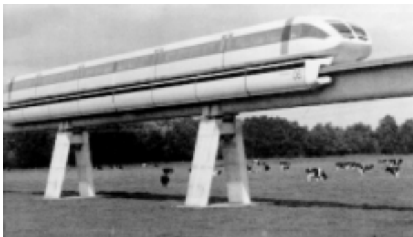
Fig. 2. TRANSRAPID 06 at EMSLAND Test Track in Northern Germany [3]
