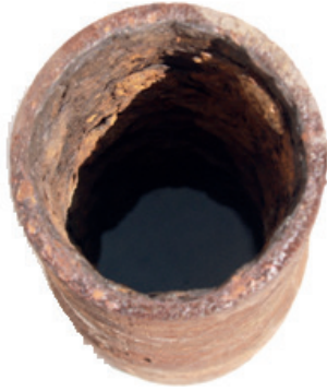
Figure 1 General corrosion of well pipes
