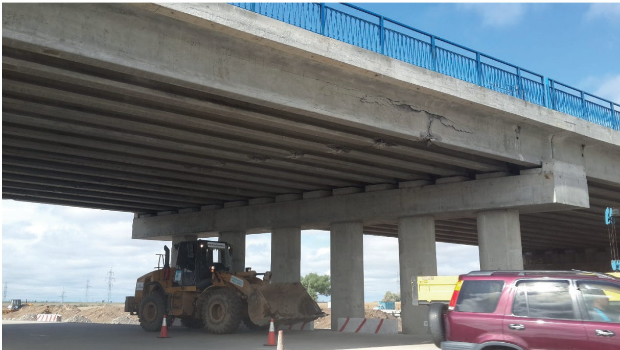
Figure 1 General view of the overpass from Kapshagai before repair
