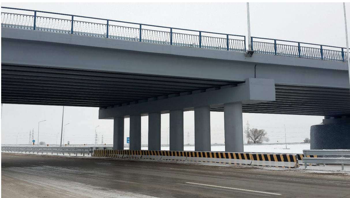
Figure 2 General view of the repaired superstructure No. 1 from Almaty
