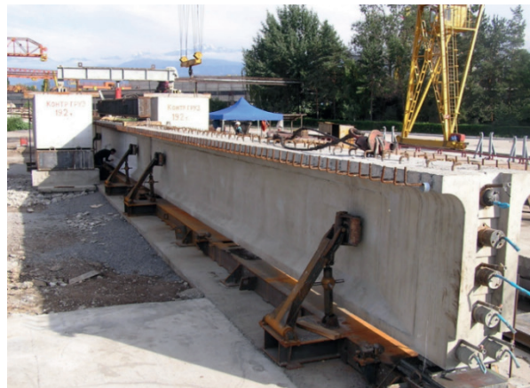
Figure 10 The fittings designed for injecting grout are shown at the end of the composite beam
