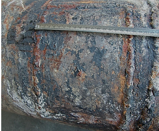
Figure 1 Steel repair-patch A
