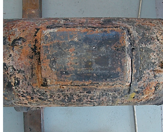
Figure 2 Steel repair-patch B
