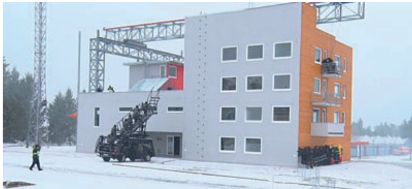
Figure 9 The northern view of the realised construction
