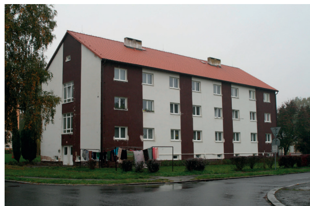
Fig. 3 The view of the pilot building in Milevsko in its present state
