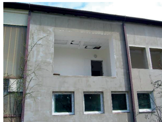
Fig. 1 Beginning of construction work on the laboratory - prepared opening for wooden frame (April 2010)
