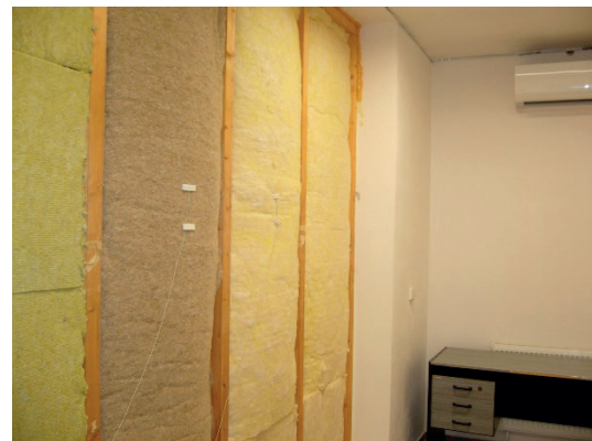
Fig. 5 Thermal insulation prior fitting vapor barrier (January 2011)
