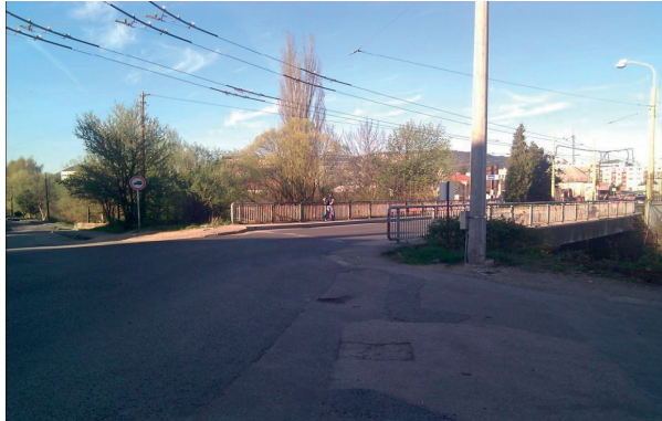
Fig. 2 Chosen bridge [authors]
