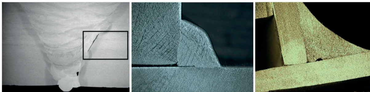
Fig. 2 Lack of fusion and penetration [4]
