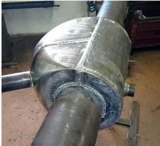
Fig. 1 Split sleeve for branch connection repairs
