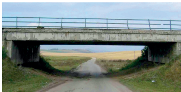
Fig. 3 The view of bridge No. 065-086 near the village Mosovce
