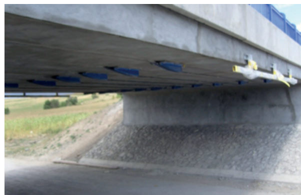
Fig. 10 Bridge No. 065-086 after strengthening by external prestressing
