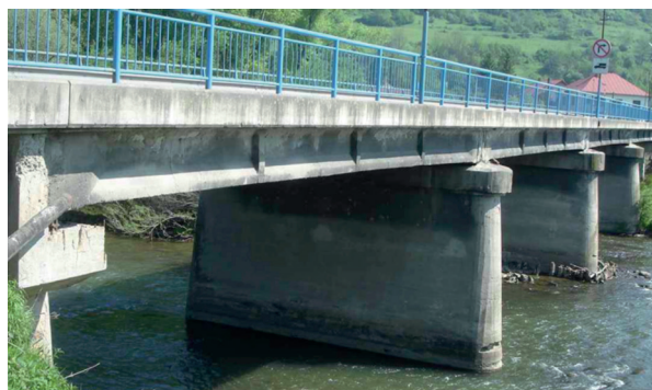
Fig. 2 The view of bridge No. 059-091 in Nizna over the river Orava
