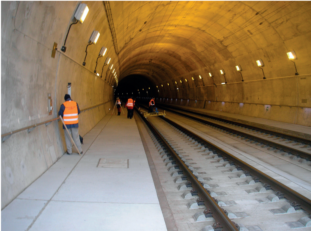
Fig. 1 View of the slab track structure in the tunnel Turecký vrch
