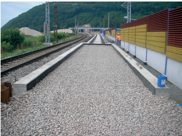
Fig. 7 View of the transition area built between the structure of the slab track and track section with standard structure of railway superstructure (left in the area of south portal and right in the area of north portal)
