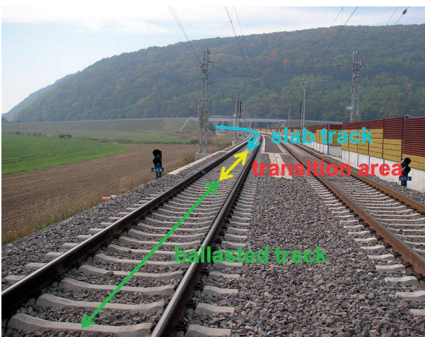
Fig. 8 View of the transition area built between the structure of the slab track and the standard structure of railway superstructure
