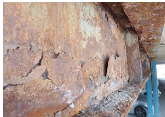
Fig. 3 Views of the steel frame details of the external car park roof structure (the condition before the renovation)
