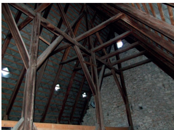
Fig. 2 View into the truss space
