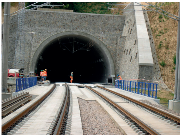
Fig. 2 Ballast-less track above the railway bridge
