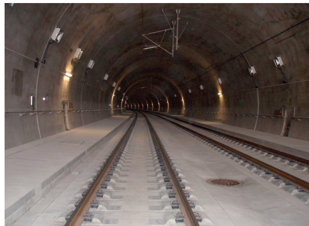
Fig. 1 Ballast-less track structure in the tunnel
