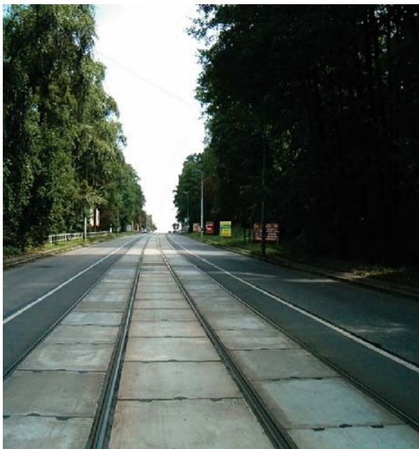
Fig. 1 Tramway track with concrete panels cover
