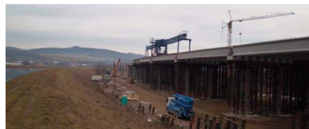
Fig. 7 Construction of the highway bridge 207
