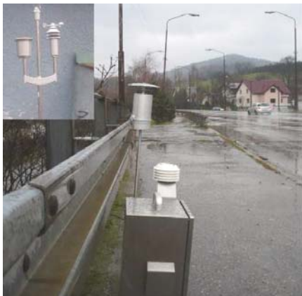
Fig. 8 Measurement at the roadway position 4 Dolny Hricov (on the left)
