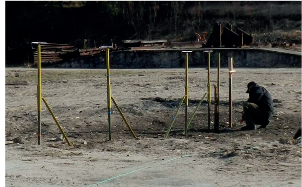
Figure 5 Preparation of measuring sensors for field tests
