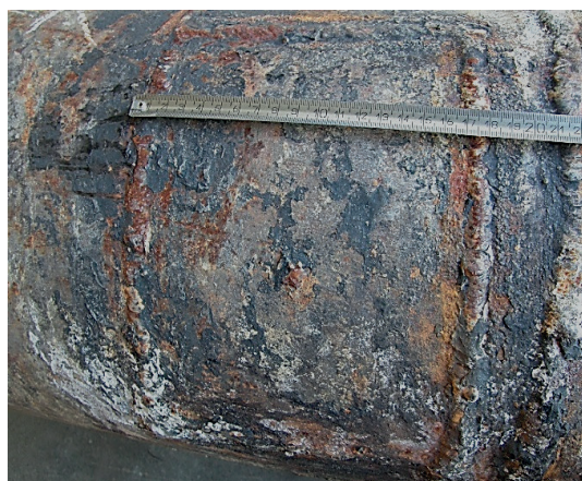
Figure 1 Steel repair-patch A
