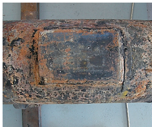
Figure 2 Steel repair-patch B
