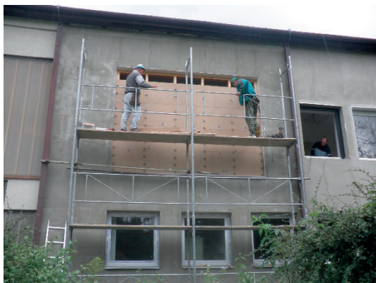
Fig. 3 Montage of MDF board (September 2010)
