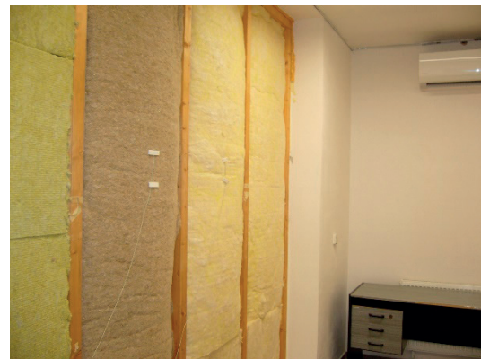
Fig. 5 Thermal insulation prior fitting vapor barrier (January 2011)
