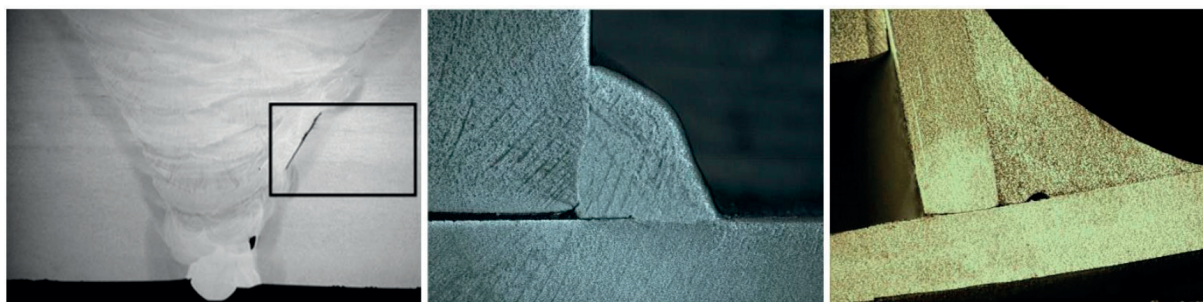
Fig. 2 Lack of fusion and penetration [4]
