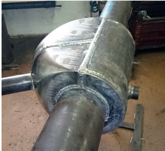
Fig. 1 Split sleeve for branch connection repairs
