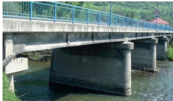
Fig. 2 The view of bridge No. 059-091 in Nizna over the river Orava
