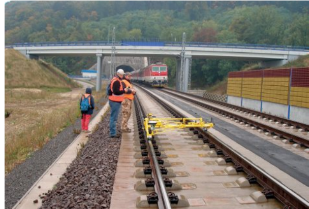
Fig. 1 Type of Ballastless Track Construction RHEDA 2000
