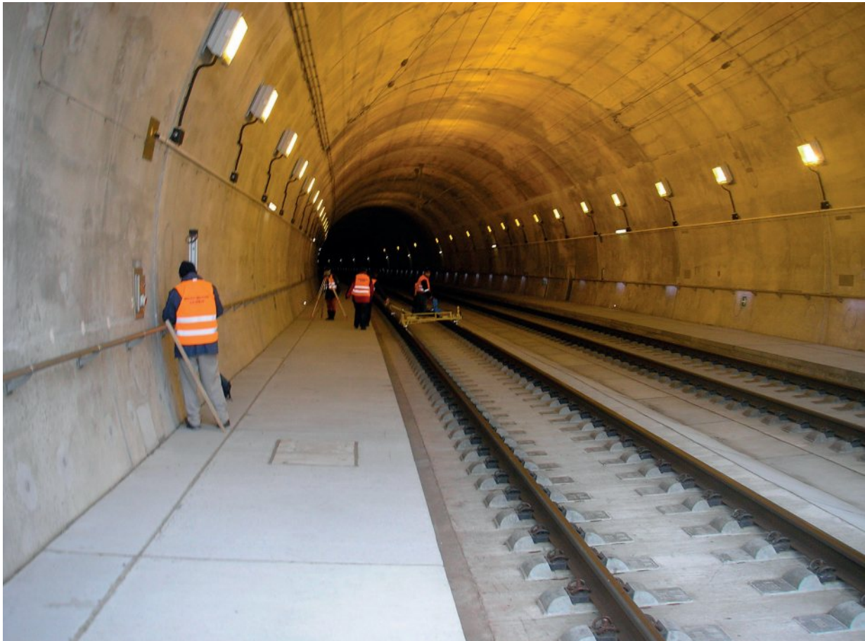
Fig. 1 View of the slab track structure in the tunnel Turecky vrch
