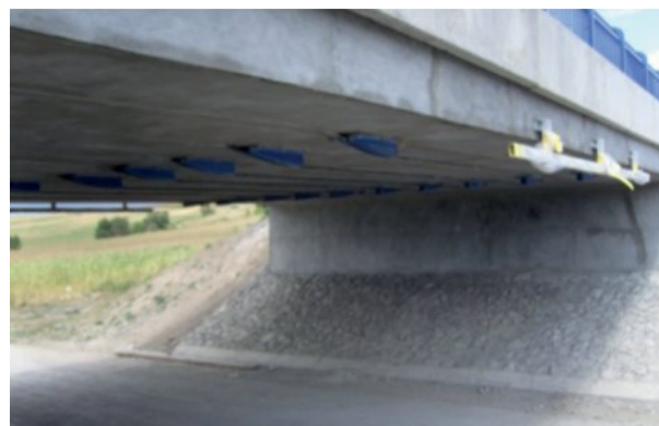
Fig. 10 Bridge No. 065-086 after strengthening by external prestressing
