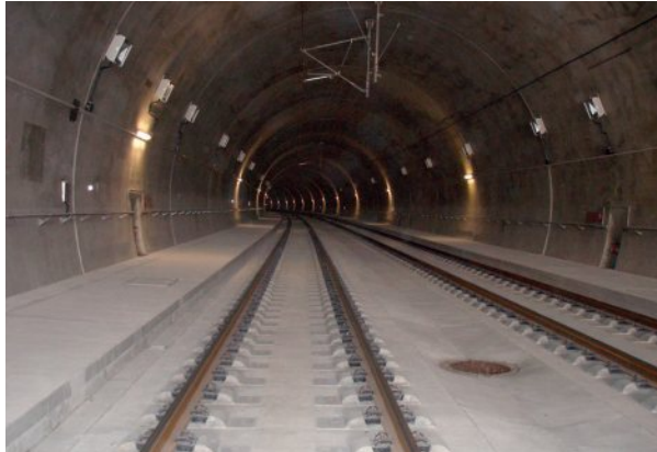
Fig. 1 Type of Ballastless Track Construction RHEDA 2000
