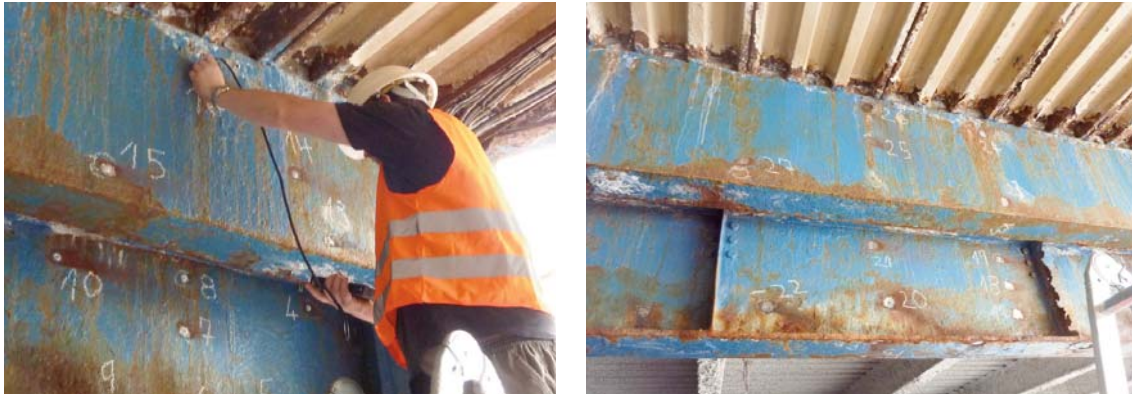
Fig. 2 Experimental measurements of the section thickness of Beam 6 in the most exposed locations
