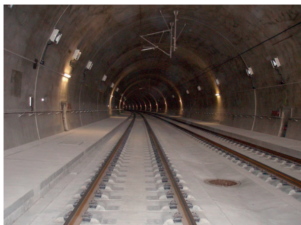
Fig. 1 Ballast-less track structure in the tunnel
