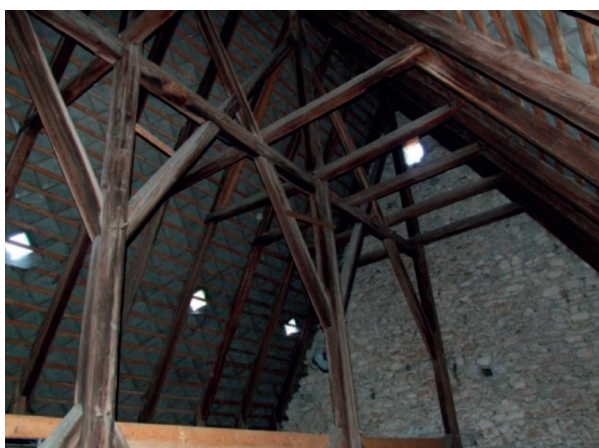
Fig. 2 View into the truss space
