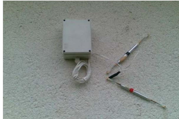
Fig. 5 Installation of a measurement unit
