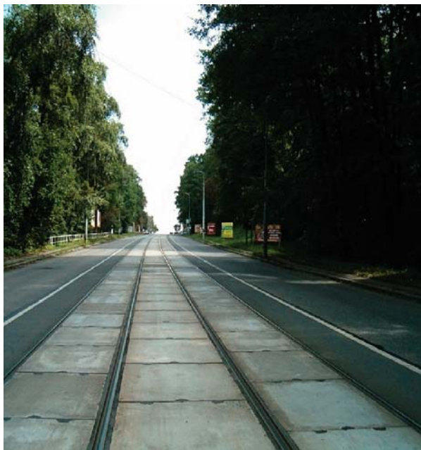
Fig. 1 Tramway track with concrete panels cover
