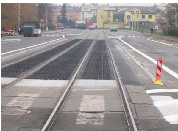
Fig. 3 The test section of the tram line with modified tiling on Zavodni street in Ostrava
