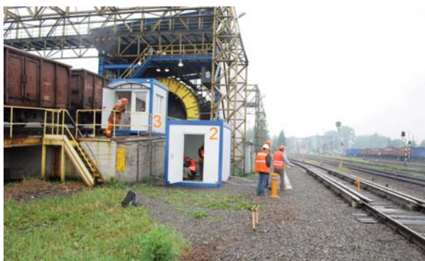
Fig. 2 Electrodynamic Wagon Retarder system at the railway siding of the Power Plant Rybnik.
