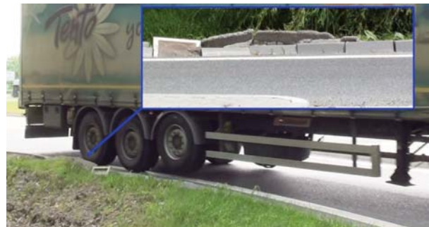
Fig. 2 Damaged right curb (roundabout VM1)
