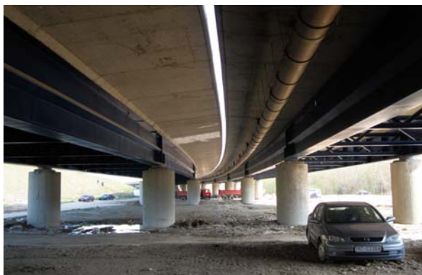
Fig. 1 View of a continuous composite bridge concrete deck
