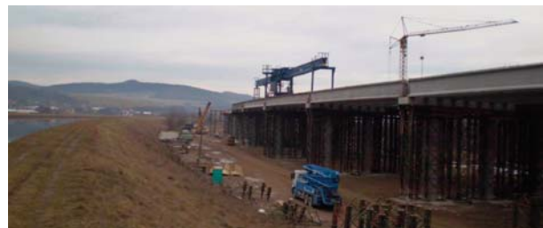
Fig. 7 Construction of the highway bridge 207
