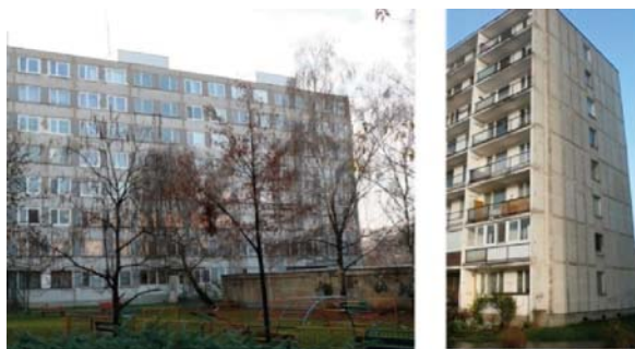
Fig. 2 Panel block of flats structural system T08B, row and solo house Kosice
