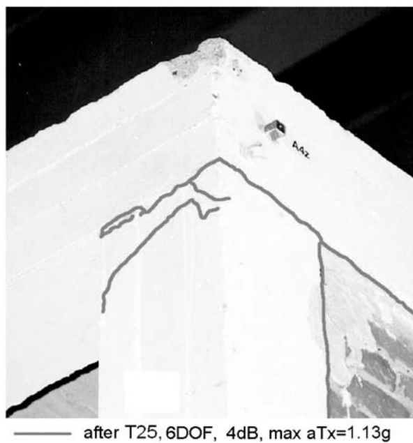
Fig. 9 Cracks in critical sections of R/C frame at the end of test - top of the frame
