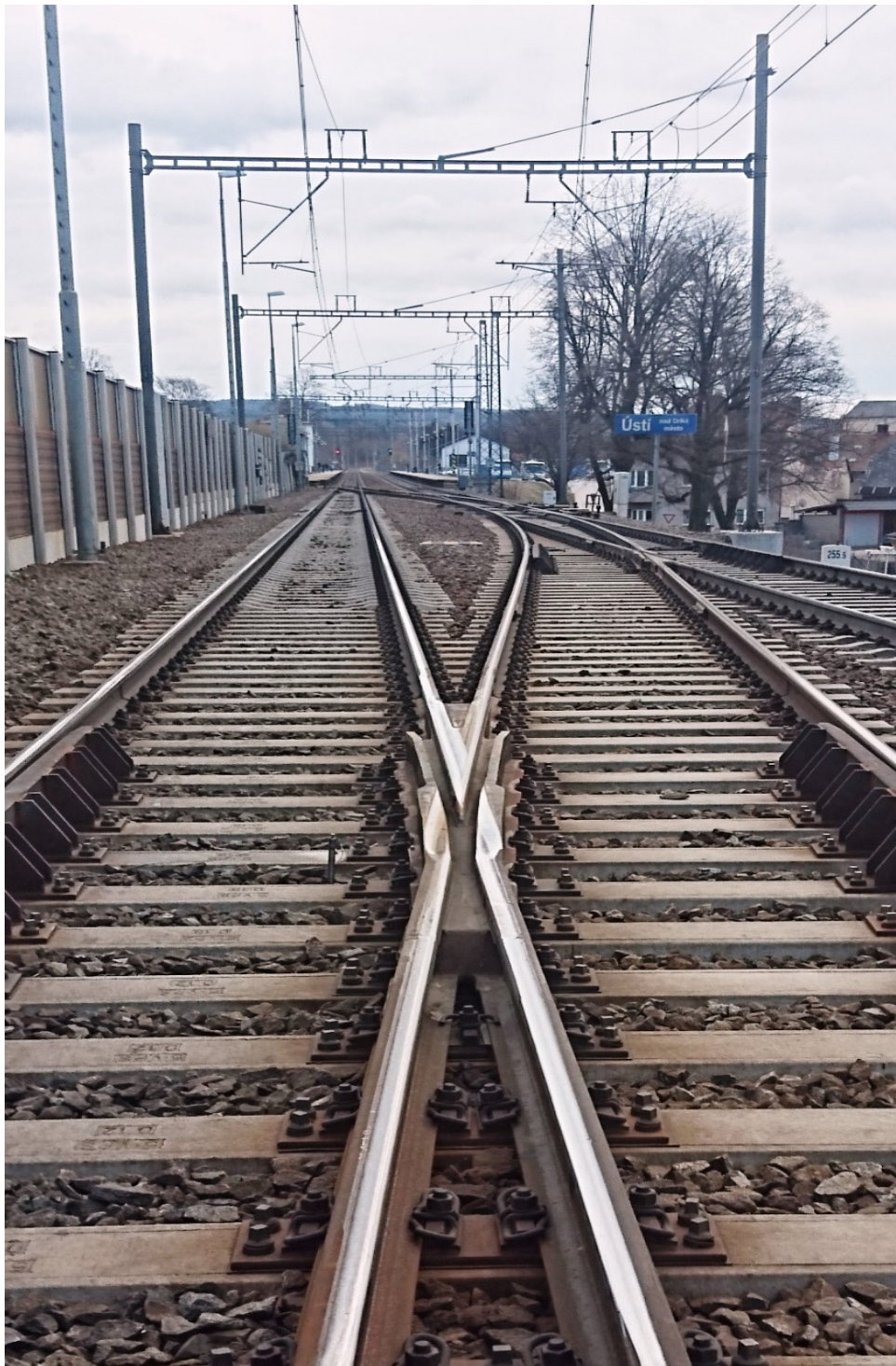
Figure 4 Measurement place, the view of switches No. 3 and No. 4
