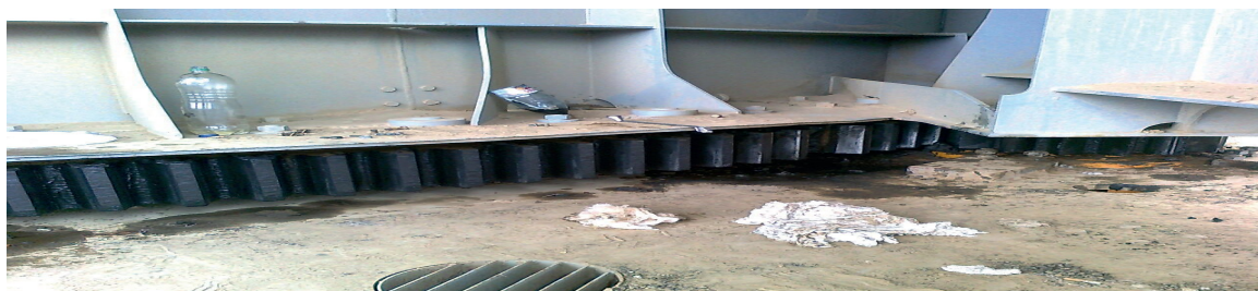
Figure 2 Appearance of the girth gear and the pinion for rotation of the excavator's upper structure
